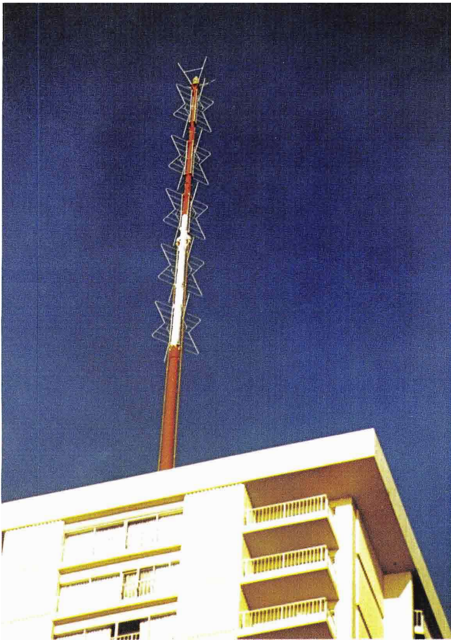
KITV's new Superturnstile Antenna atop the Ala Moana Hotel.
