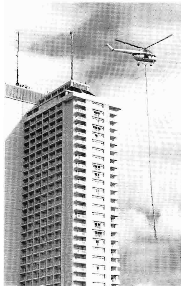
With the lower sections in place, a 3-bay section is air-lifted.
